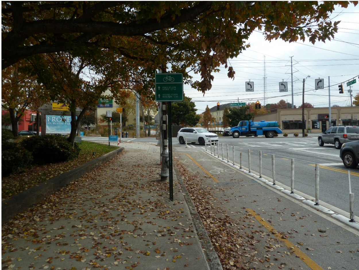
Figure 4-34. A Separated Bicycle Lane with Leaf Debris
